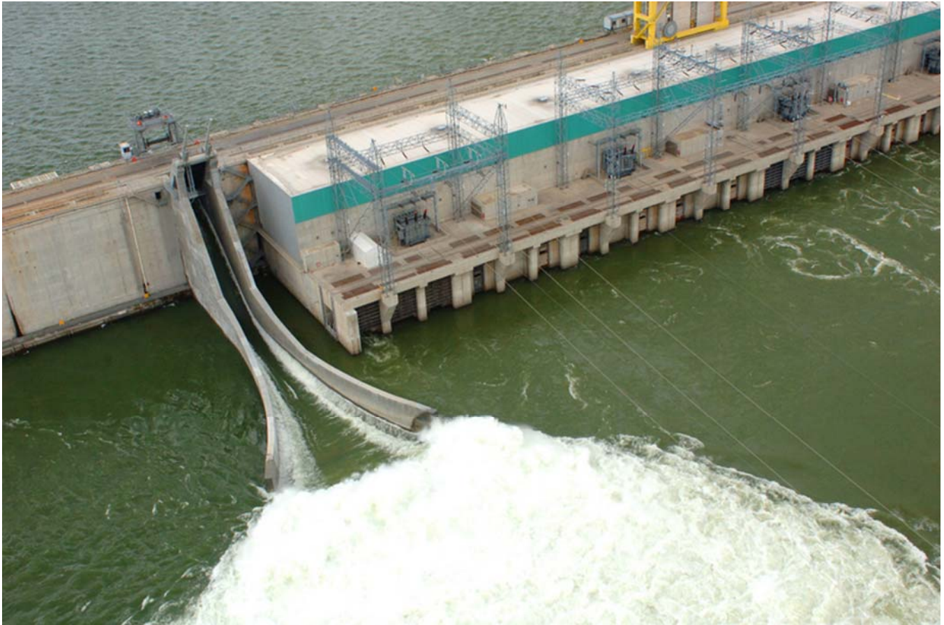
(Grant PUD Aerial Image: Wanapum Dam Fish Bypass in operation. The new bypass yielded high survival rates for fish while at the same time allowing for an increase in overall electric generation at the dam.)
